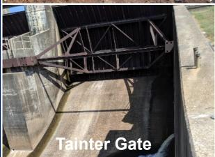
The Brazos River Authority owns and operates Sterling C. Robertson (SCR) Dam, which is located in Leon and Robertson Counties. The dam, which forms Lake Limestone Reservoir, was completed in 1978. The service spillway structure includes an overflow section with five (5) Tainter gates, non-overflow sections at the left and right sides, a stilling basin downstream, low flow outlets through the left and right end piers, and a service bridge spanning between the piers of the service spillway.
